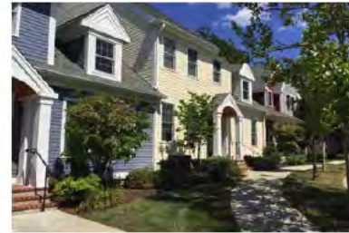
Right: Townhouses in the Red Mill Village community use variations in height, dormers, color, and type to provide visual interest and break up the larger structure. Units are designed to look like a series of attached single units.
