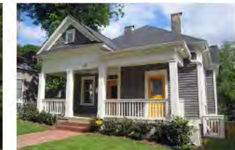
Example of a single-family house converted into a duplex. A single porch helps blend seamlessly into an existing single family neighborhood.
