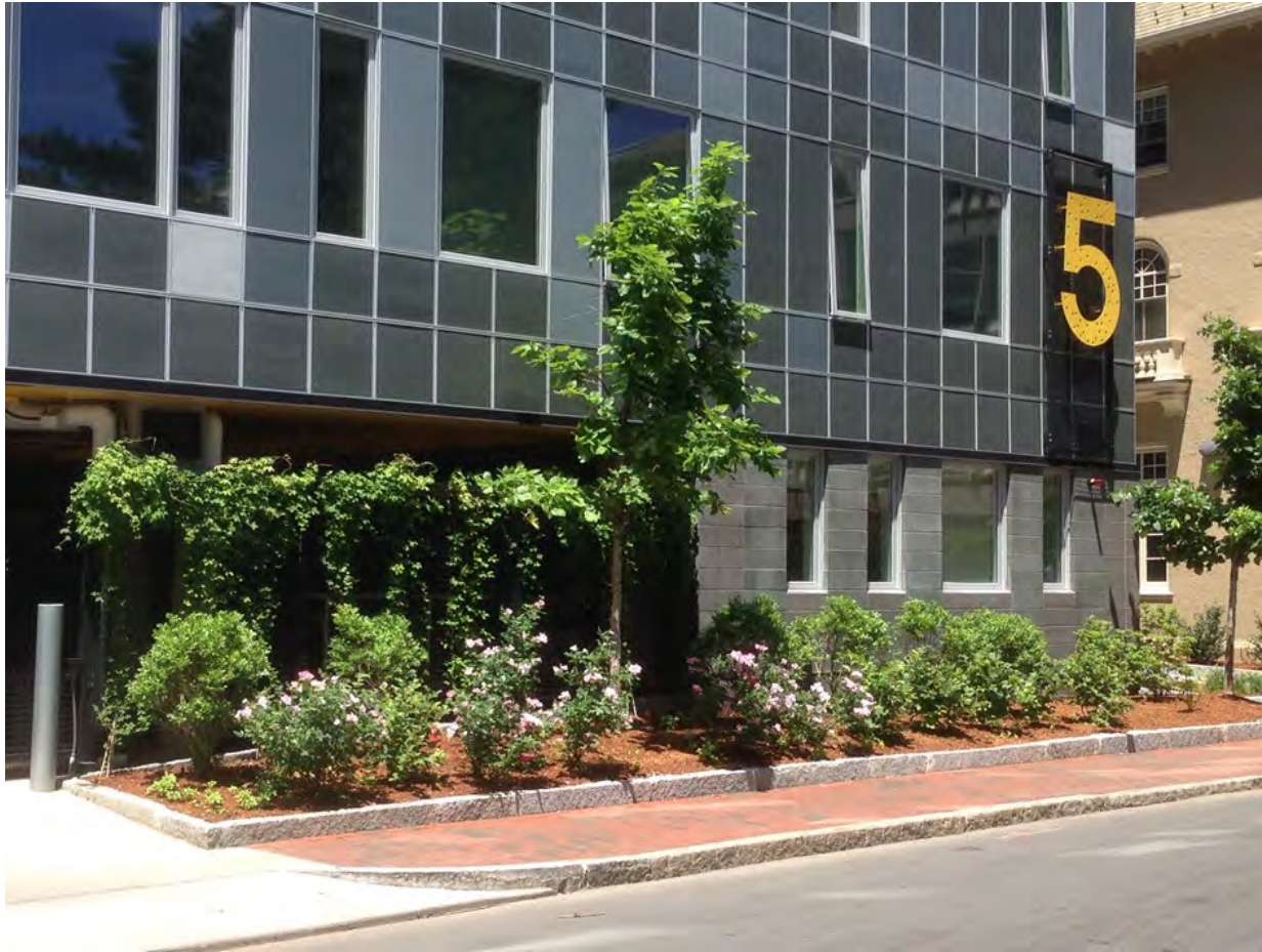
Temple Place: the comprehensive permit for this 40-unit affordable development was appealed, delaying the project for almost 3 years, and forcing a re-design of the building which resulted in the reduction of family-size units and the loss of 2 units
